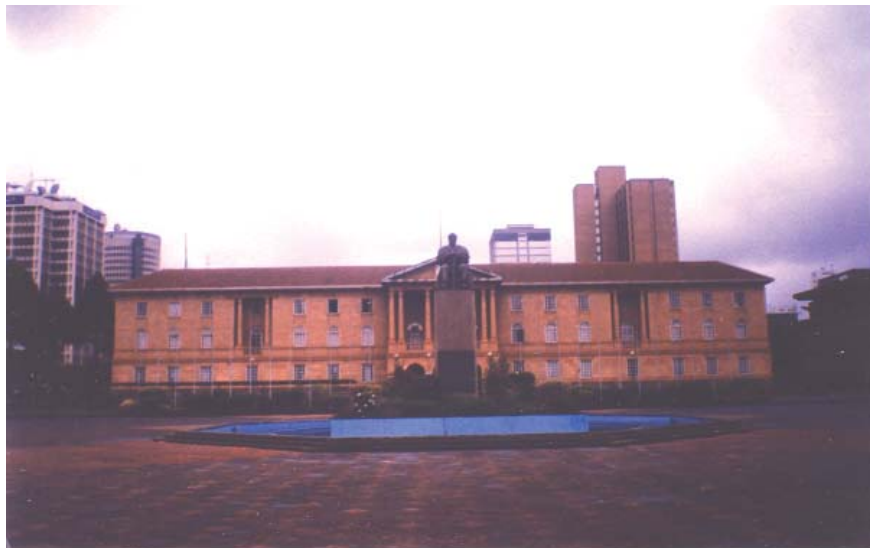
Nairobi High Court building. They maintain law and order.
